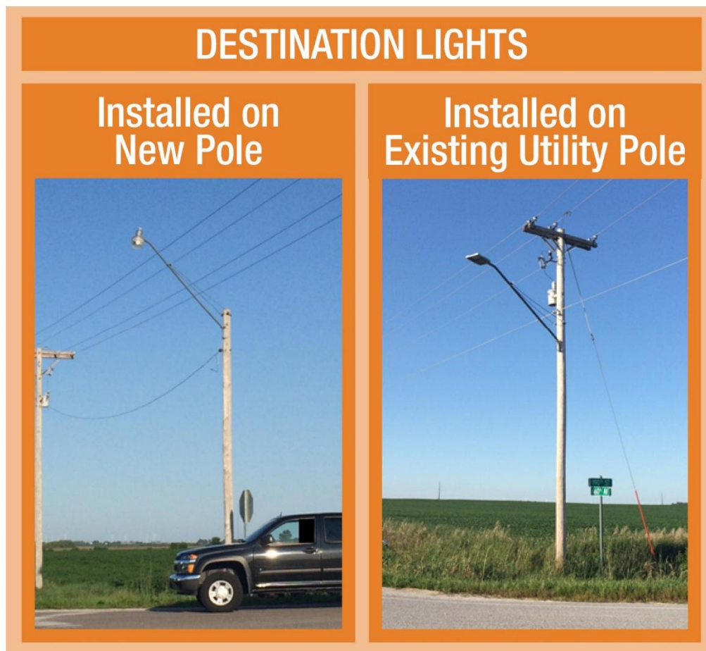
Figure 26 – Destination Lighting Installation Options
