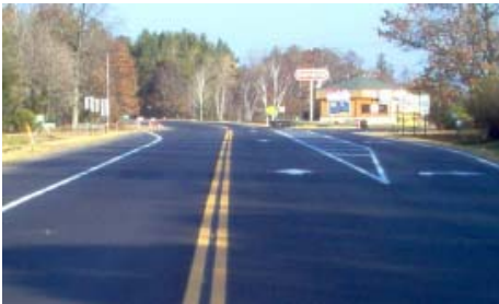
Crow Wing County, MN installed offset turn lane in a tourist area.
