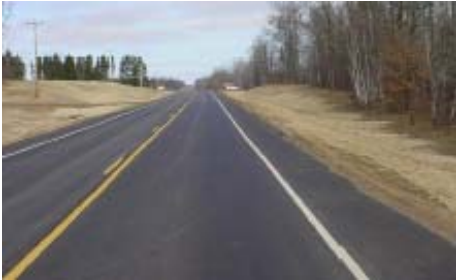
Cass County, MN paved shoulders and improved right of way.
