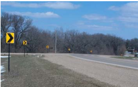
Freeborn County, MN installed chevrons along horizontal curves.
