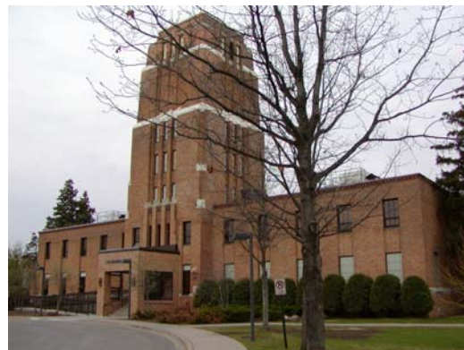
The Administration Wing of Hennepin County's Adult Corrections Facility.
