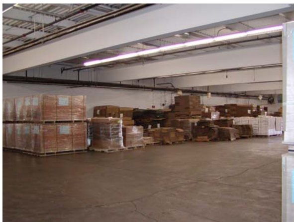
AFTER Painting: Finished Industries Warehouse with its new coat of recycled paint at the Adult Corrections Facility.
