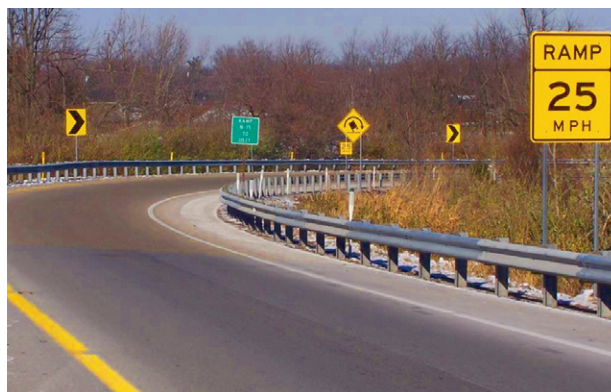
Twenty-eight percent of all fatal crashes occur on horizontal curves. Chevron signs send a strong visual cue to slow down.
