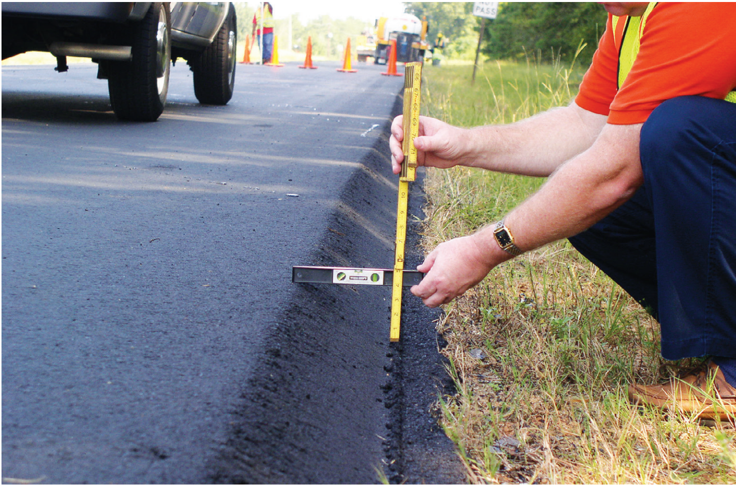
Paved and sloped safety edges can make it easier for a vehicle that has left the roadway to return to the pavement.
