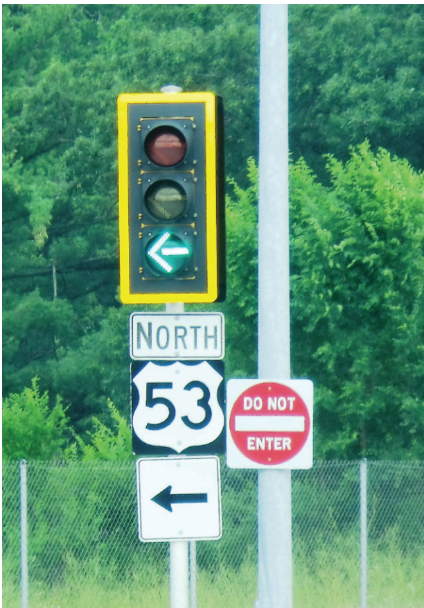
Traffic signals are easier to see, especially in bright sunlight, if they have back plates. At night, headlights cause the yellow border to reflect light back to the driver.
