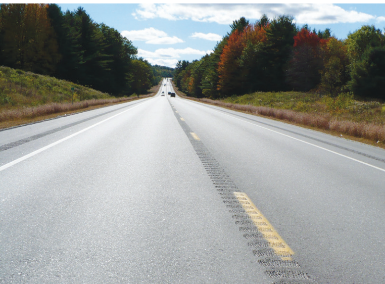
Centerline rumble strips on rural two-lane roads can reduce head-on or fatal-injury crashes by up to 44 percent.
