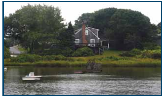
CanVis: After Structures Added
