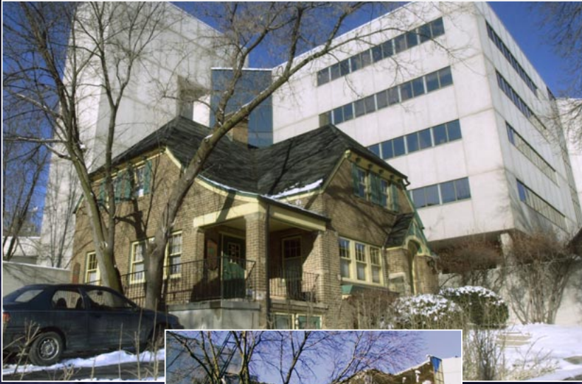
site before deconstruction
