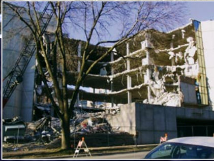
deconstruction in progress
