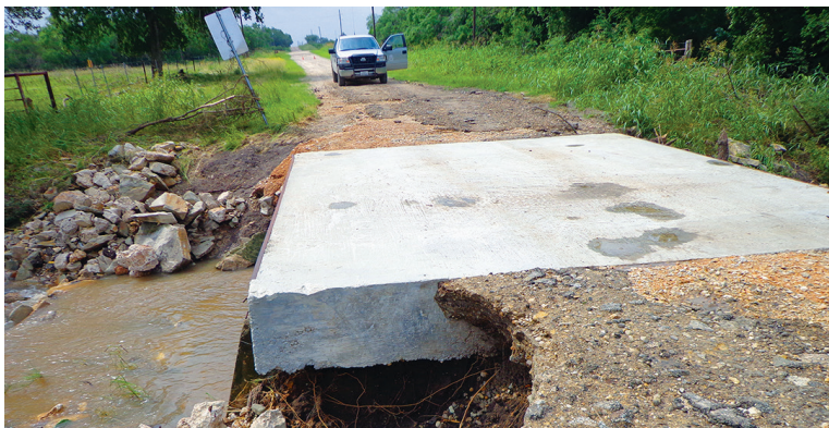
The Rakowitz Bridge in Wilson County, Texas has been judged to be structurally deficient, following May flooding, but trucks are removing barricades and crossing it anyway.
