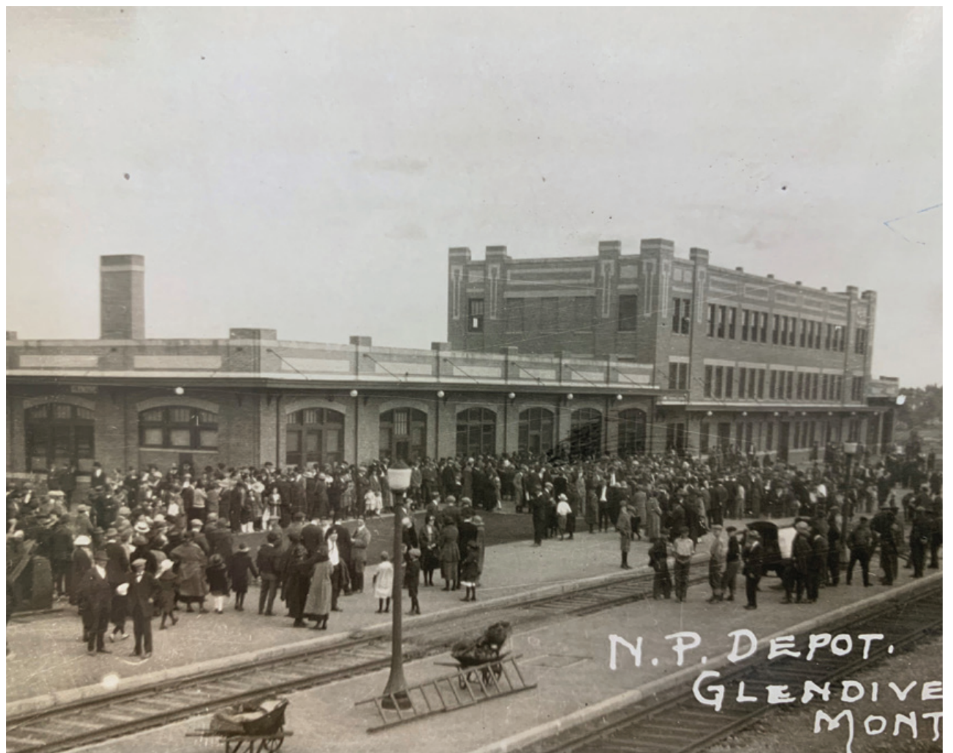
People wait at the former Glendive, Mont. passenger rail depot in Dawson County. Part of the depot still exists and is in use by BNSF Railway. Photo courtesy of the Dawson County Economic Development Council
