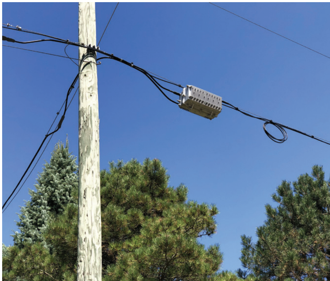
A fiber optic "node" is capable of providing gigabit speed data services to hundreds of homes.
