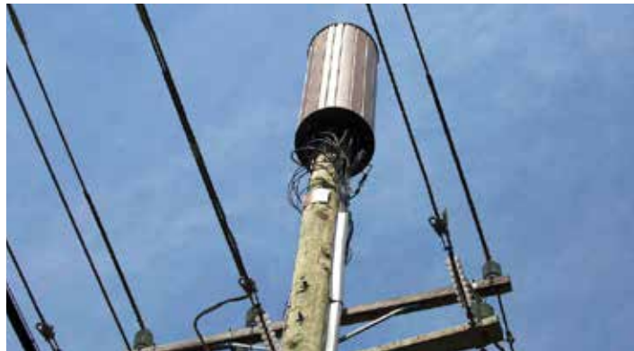
5G equipment installed above power lines. Photo by Denny Gainer
