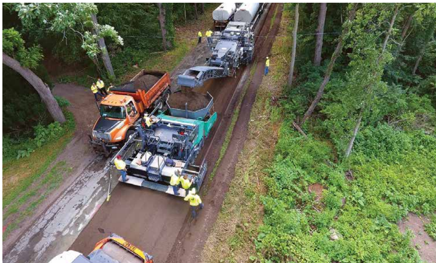
Crews use The Wirtgen 3800 recycler to recycle a road in Jackson County.
