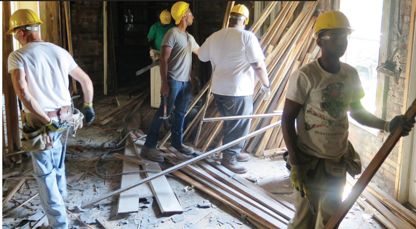
Revive Pontiac deconstruction trainees in Oakland County, Mich. get hands-on experience in how to reclaim resusable building elements that can be sold as architectural salvage. Such sales will help sustain the program. Photo courtesy of Oakland County, Mich.
