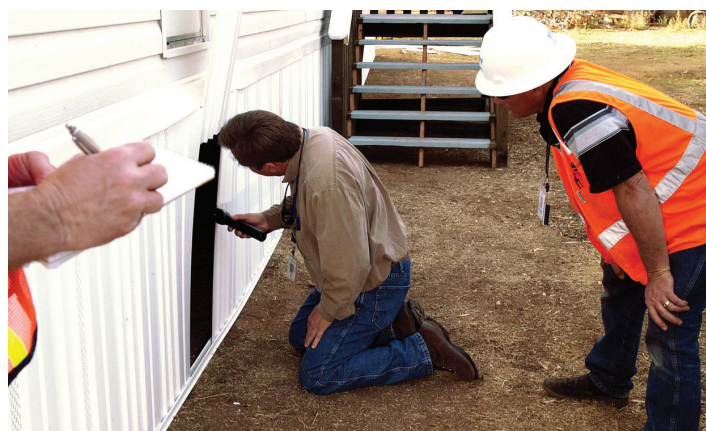
A San Diego County, Calif. building inspector checks the piers supporting a mobile home to ensure the work complies with local building codes and ordinances. Photo by Amanda Bicknell/FEMA
