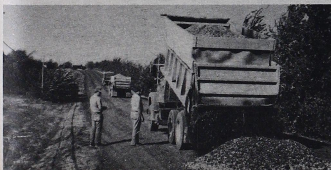
Jackson County (Mo.) experiments with a cold asphalt recycling project.
