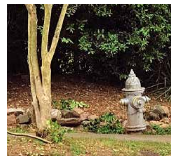
This fire hydrant connects two aging water mains contributing to low water pressure. Photo courtesy of DeKalb County
