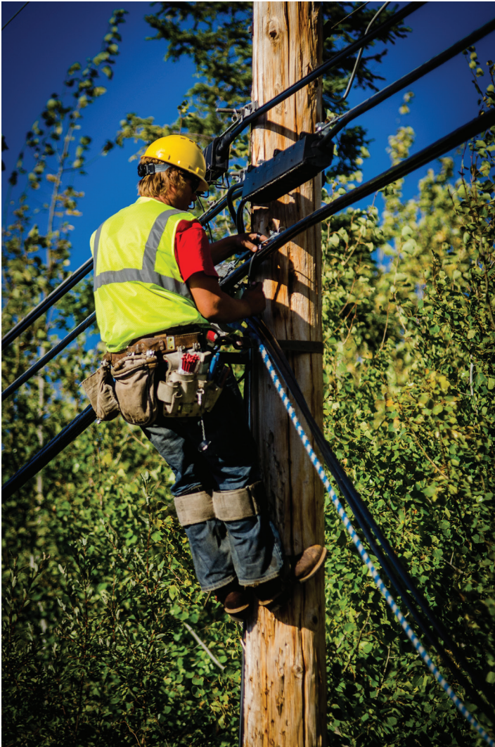
A contract employee in Lake County, Minn. attaches fiber-optic cable that comprises the above-ground portion of Lake Connections, a county-owned broadband provider. The majority of the system is underground. Photo courtesy of Lake County, Minn.
