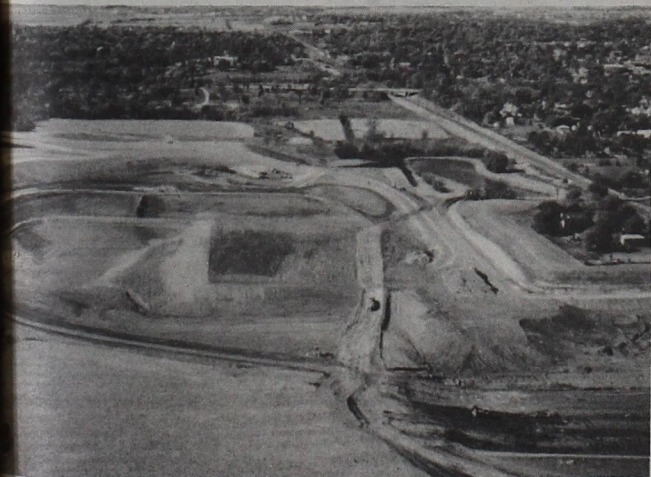
Occupying approximately 400 acres, the Settler's Hill landfill is a state-of-the-art disposal site equipped with leachate and gas collection systems. Methane gas recovered from the facility powers generators which supply electricity to Waste Management, of North America, Inc.'s nearby Environmental Monitoring Laboratories, as well as to 7,000 area residents.
