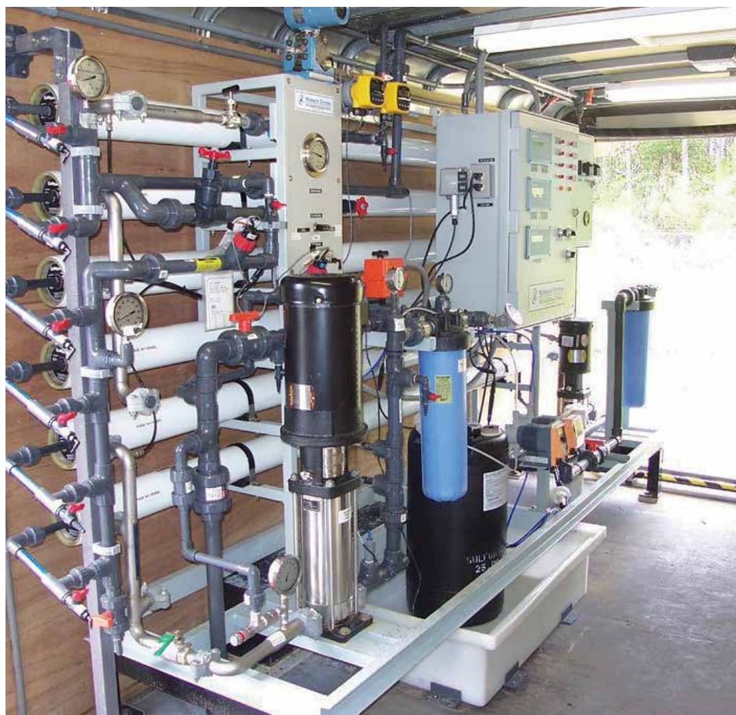
Brunswick County, N.C. is using a low-pressure reverse osmosis system to filter PFAS chemicals from the Cape Fear River. This scaled-down model was tested in 2018. Photo courtesy of Brunswick County
