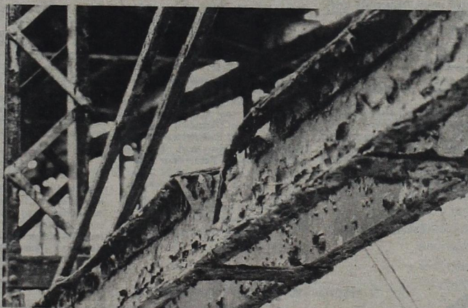
WEIGHT LIMIT IGNORED —Sanilac County, Mich., with 187 bridges on its county road system, faces a bill of $120,000 to replace the bridge at left. Although it was posted with a 10 ton weight restriction, enforcement is extremely difficult on all 187 bridges. This 10-ton truck was carrying approximately 16 tons of pickles. The county intends to sue the local farmer who lives a half mile from the bridge.
