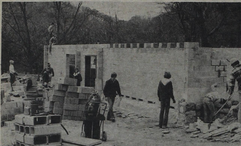
"Vo-tech" students are doing the masonry block work and 90 per cent of the electrical wiring for the center.
