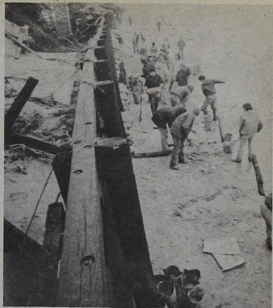
Suffolk County Conservation Corps crews working feverishly against a rising tide and wind-whipped rain to sandbag a damaged bulkhead on a Rocky Point beachfront.
