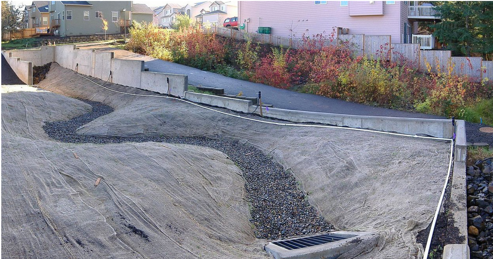
Two bioswales: One in the foreground under construction and before landscaping. The background, vegetated swale is completed. This green infrastructure captures polluted storm water rushing off hard surfaces like parking lots, roads, driveways and rooftops. Other types of green infrastructure retrofits include downspout disconnection — rerouting rooftop drainage pipes to rain barrels, cisterns or permeable areas instead of the storm sewer. Image from the Wikimedia Commons, released into the public domain by the author.
