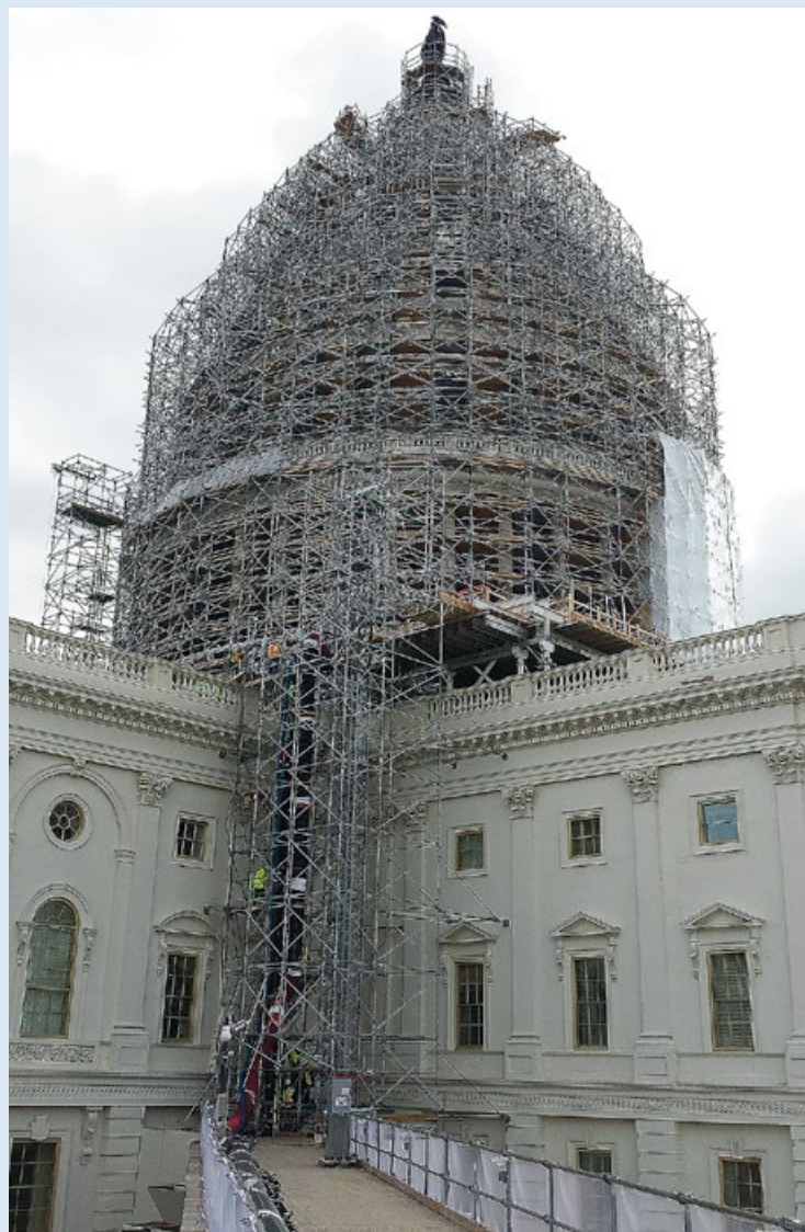
Infrastructure needs get a boost on Capitol Hill. Scaffolding encases the U.S. Capitol dome as workers begin to repair more than 1,000 cracks on the 149-year-old iron structure. If laid end-to-end, the scaffolding would be 52 miles long.
