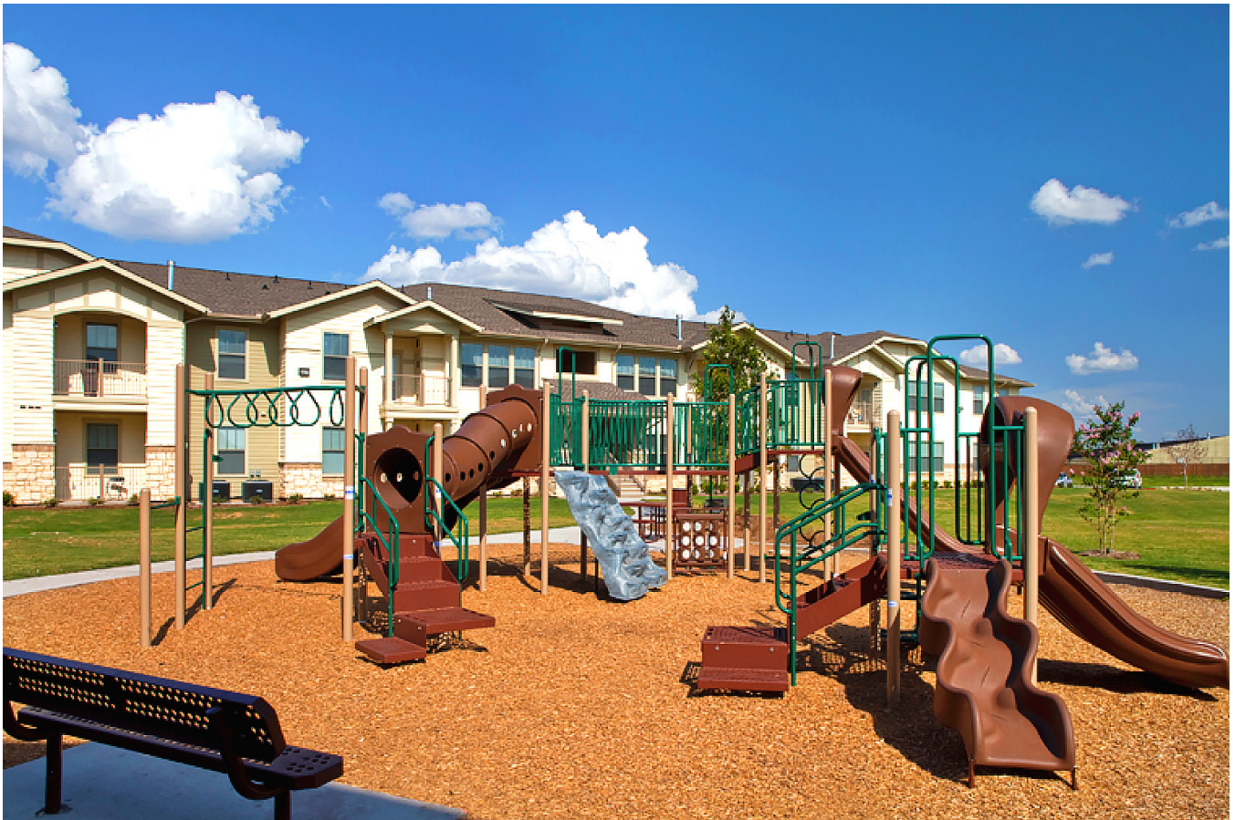
Costa Esmeralda Apartments in McLennan County, Texas is a 112-unit LITHC family development built in 2011 and managed by THF.
