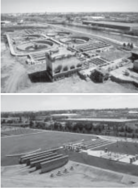
North Denver's 70-acre Northside wastewater treatment plant (top) along the South Platte River was polluted by multiple contaminants. An extensive partnership led by the City and County of Denver redeveloped the abandoned sewage plant into a new 13-acre park, a wetland, a storm water retention pond, and a National Guard Armory — a good example of brownfields redevelopment.
