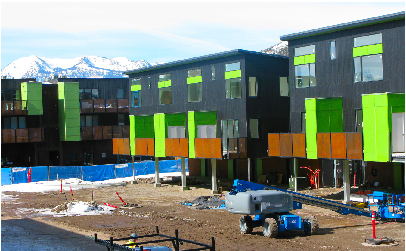
Teton County (Wyo.) apartment and condo-style affordable housing units for employees.
