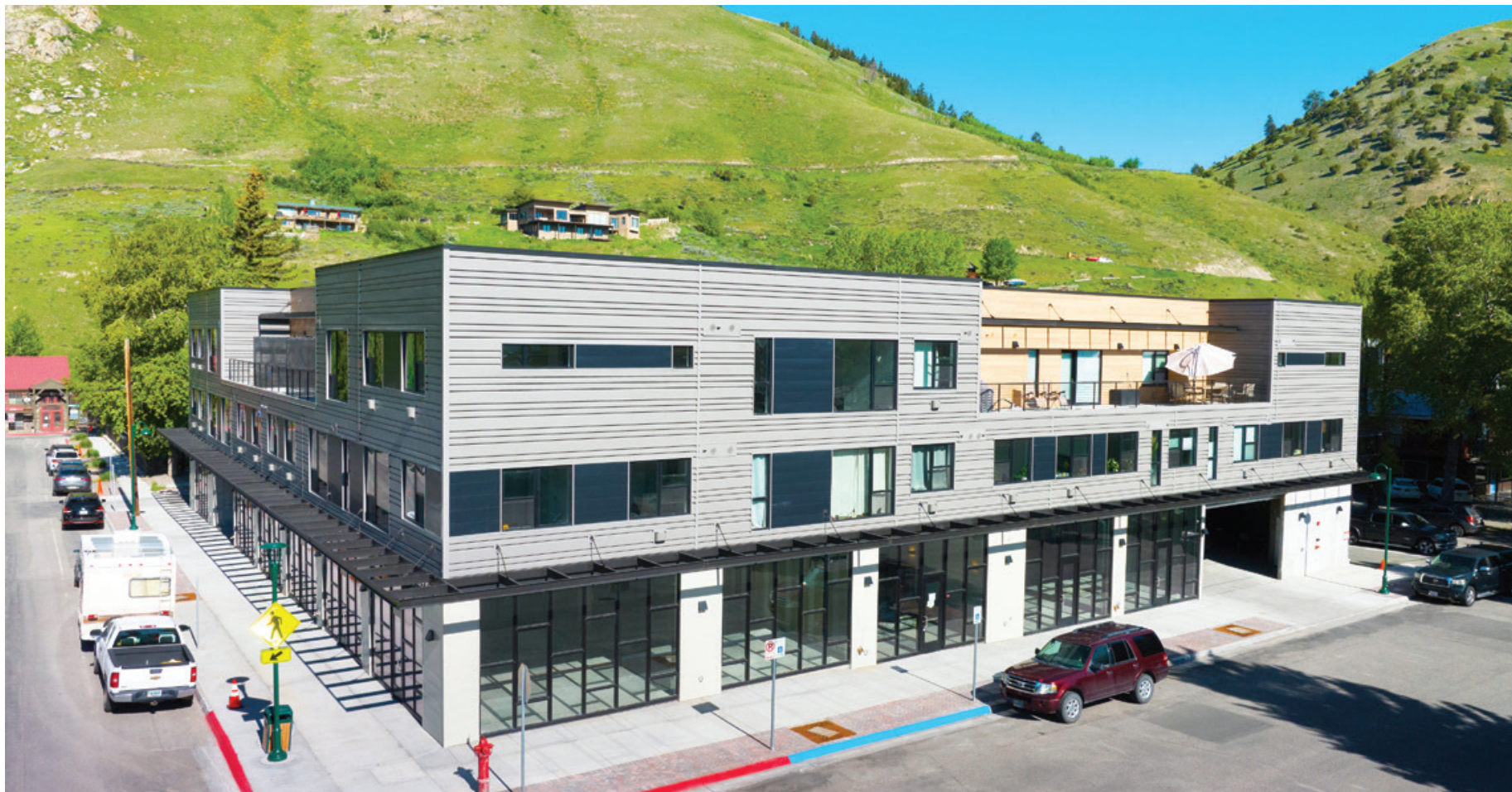
Teton County worked with Mercill Partners to create 30 workforce condominiums, 20 one-bedroom homes and 10 two-bedroom homes. Photo courtesy of April Norton
