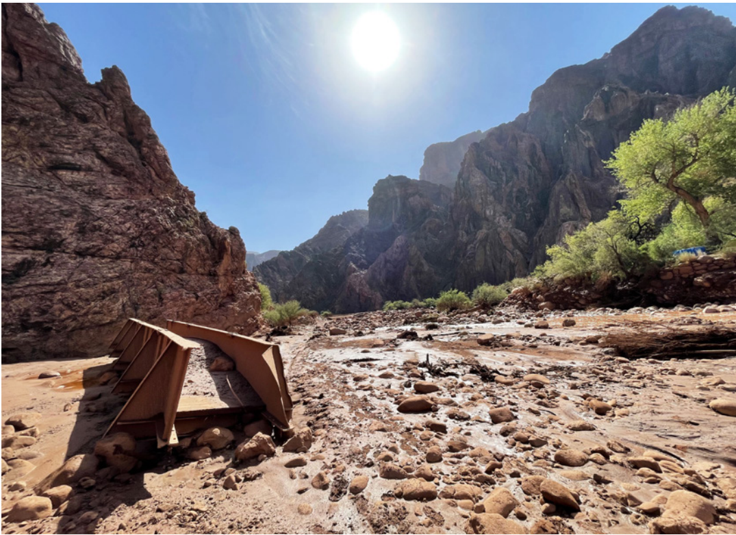
A footbridge lies along Bright Angel Creek in Grand Canyon National Park after it was washed away during the Aug. 29 Colorado River flash flood. Photo courtesy of the National Park Service
