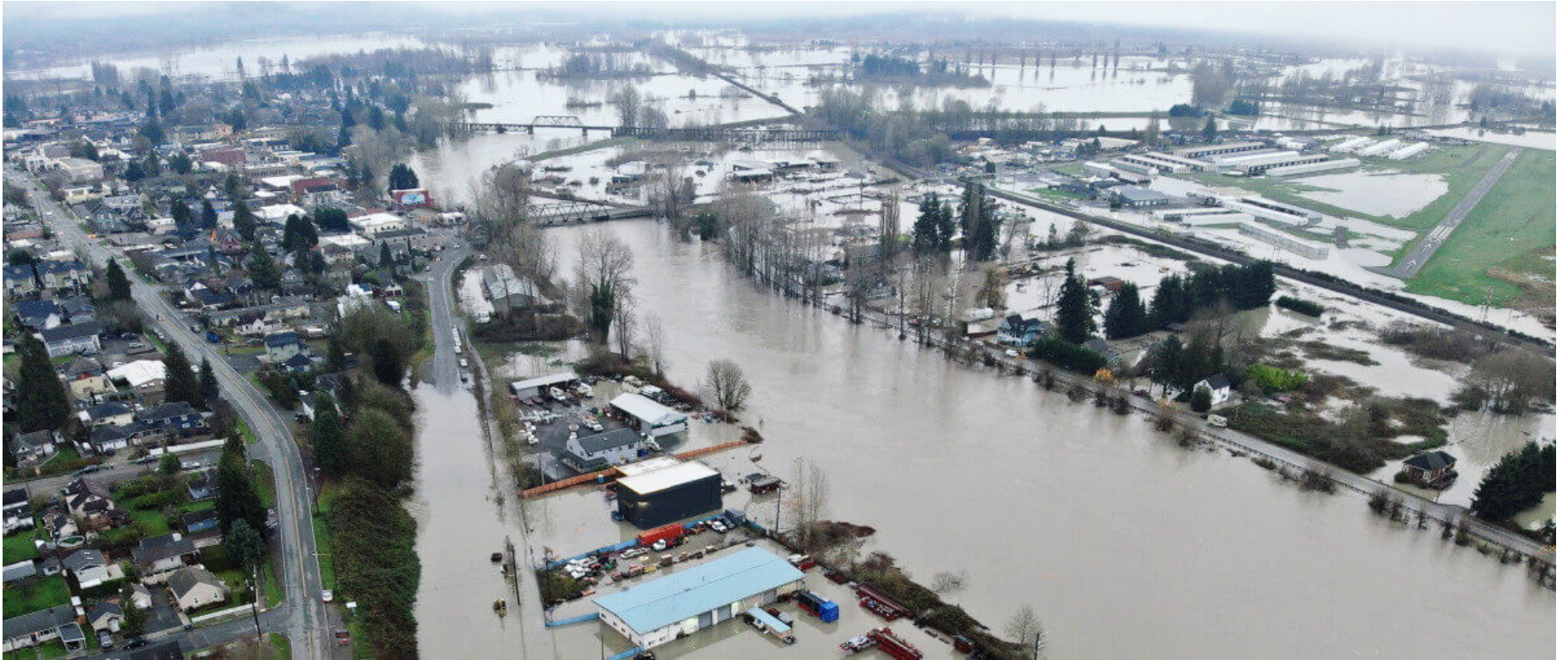
A powerful atmospheric river causes widespread flooding across Washington state in December 2025, damaging homes, businesses and major roadways.
