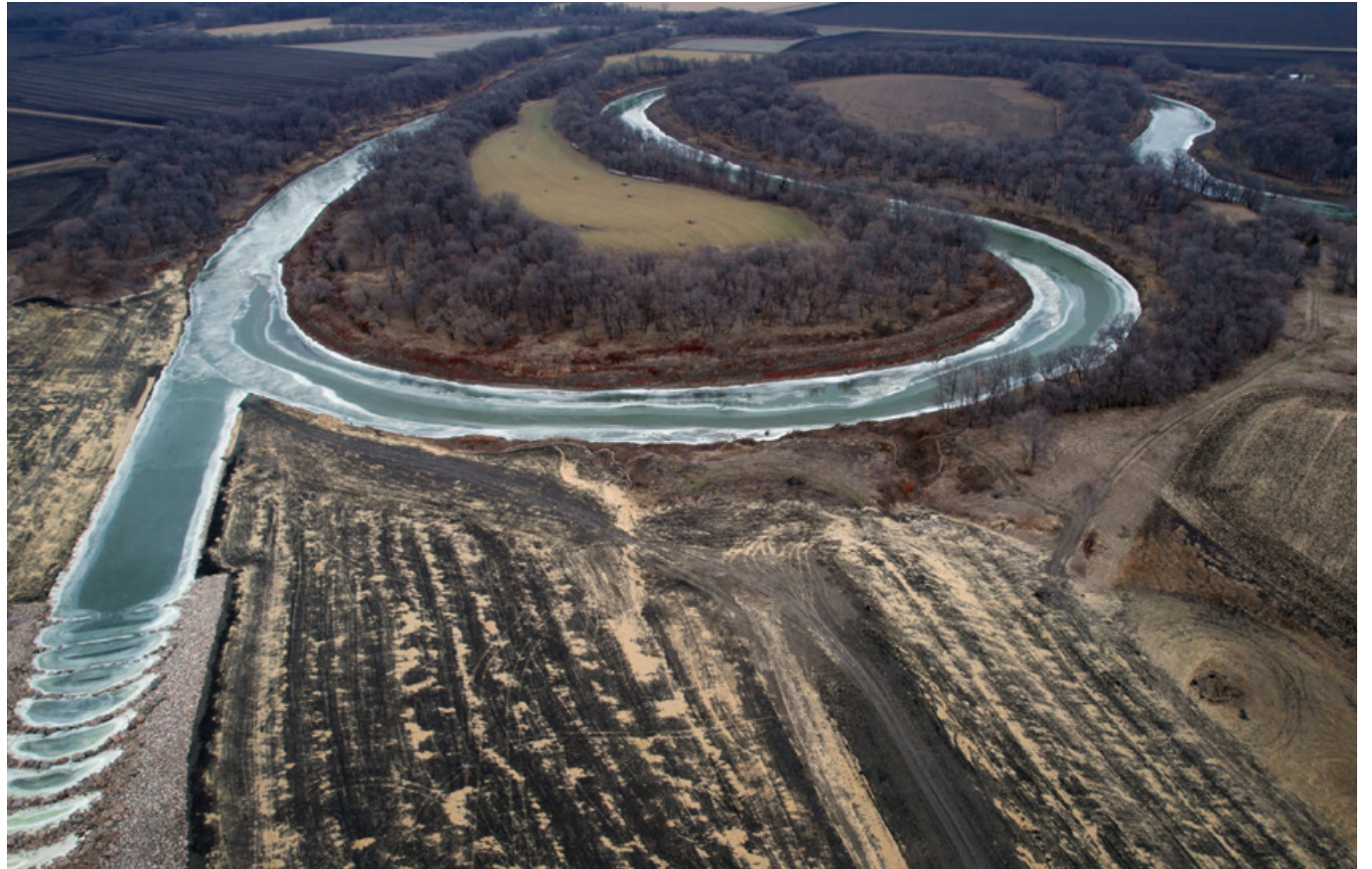
A diversion outlet returns floodwaters to the Red River in northern Cass County, N.D. A diversion channel carries floodwater west of Fargo and other Cass County areas. Photo courtesy of the Army Corps of Engineers
