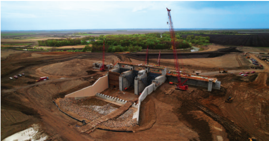
This diversion inlet will collect flood waters on the Red River south of Fargo and redirect to the west, around developed areas, and back to the river. Photo courtesy of the Army Corps of Engineers
