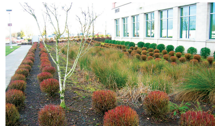
Shrubs can draw in more rainwater diverted from roofs and other impervious surfaces. Photo courtesy of Clackamas County, Ore.
