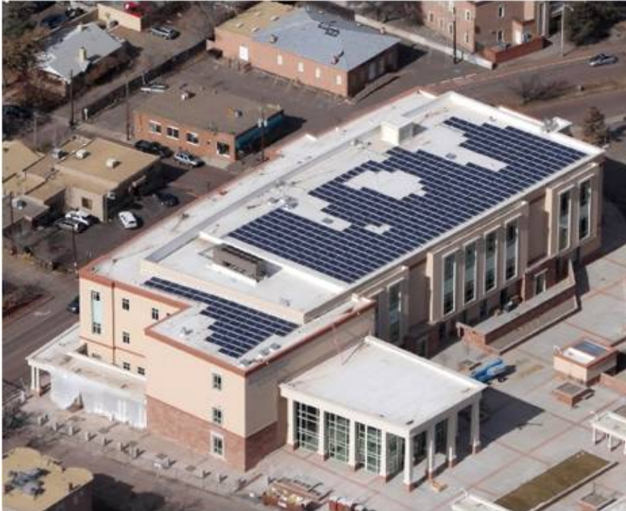
New County Courthouse 113 kW PV System – 20% Of Electric Needs
