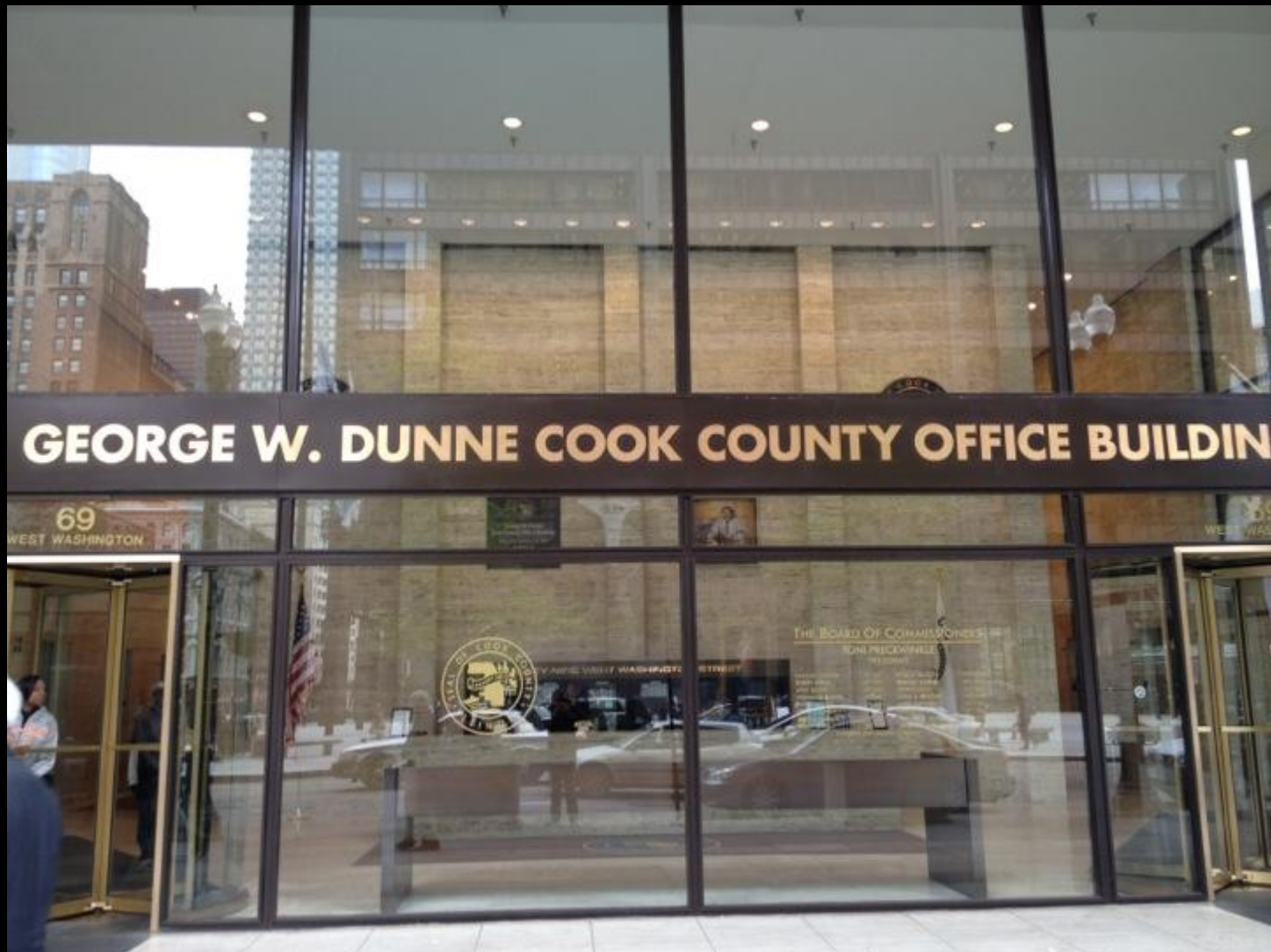
George W. Dunne Cook County Office Building: ENERGY STAR Certified 2008-2012
