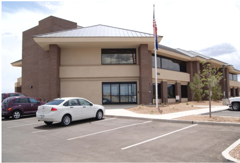
Mohave's Development Services Building (above) is the 2 nd LEED certified building in northwest Arizona and features a sustainable cooling system.
