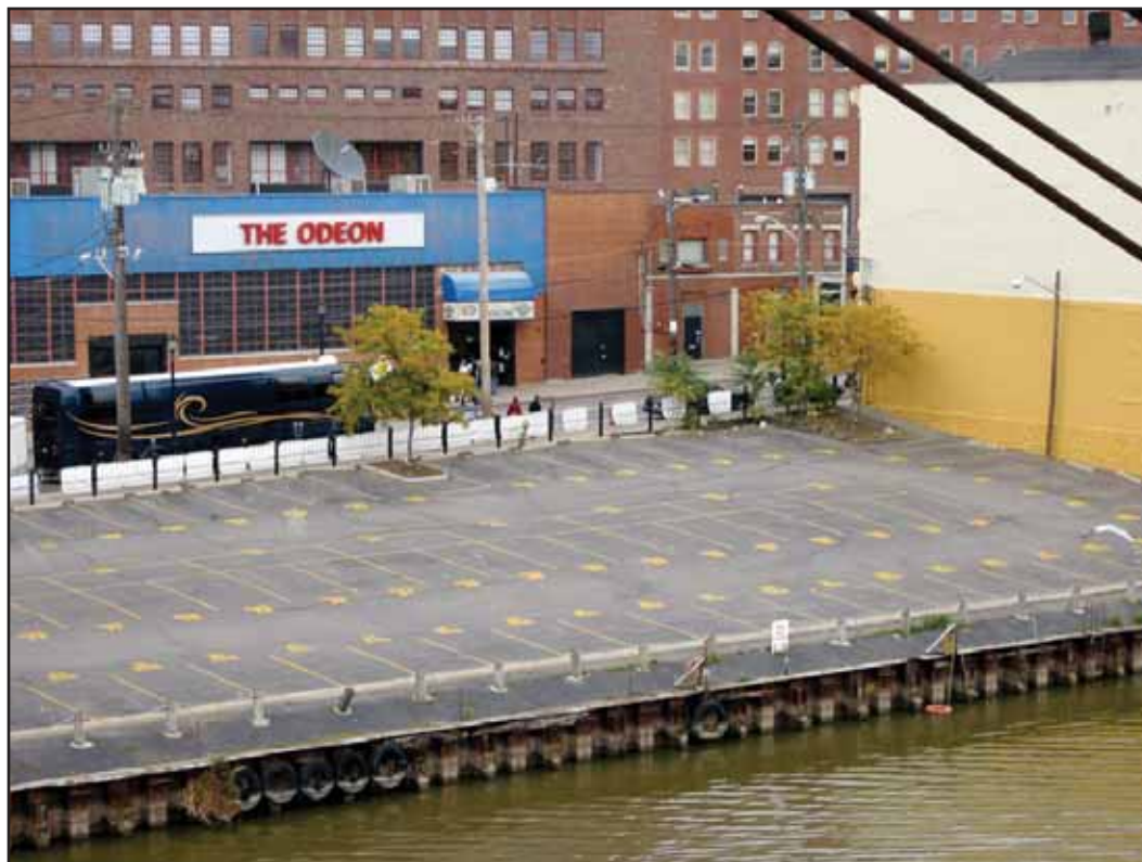
Impermeable surfaces like this parking lot in downtown Cleveland create stormwater runoff that can subsequently pollute waterways.
