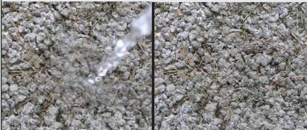
A porous pavement trail at Lakewood Park absorbs water that otherwise would run off.
