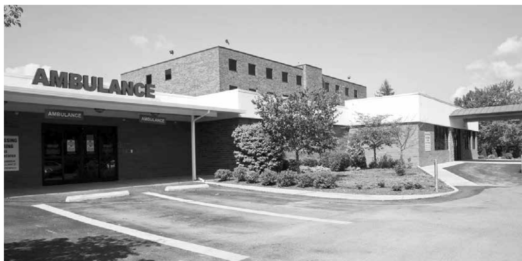
Lee County (Va.) Regional Medical Center closed in 2013; the county stepped in to help reopen it five years later. Photo courtesy of The Roanoke Times
