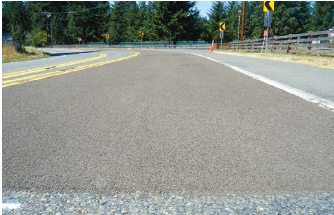
An example of curve safety treatments: high-friction surface treatment provides vehicles more traction and chevron signs warn of dangerous curves ahead. Photo courtesy of Scott Davis, Thurston County, Wash.
