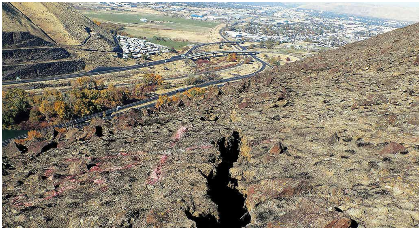
Cracks like this along Rattlesnake Ridge in Yakima County, Wash. were discovered in late October last year. Since then they have expanded and an entire hillside is sliding now at a rate of about 1.6 feet per week threatening Interstate 82, the Yakima River and communities below. See page 3 to learn more about how the county is responding. Photo by Steve Reidel
