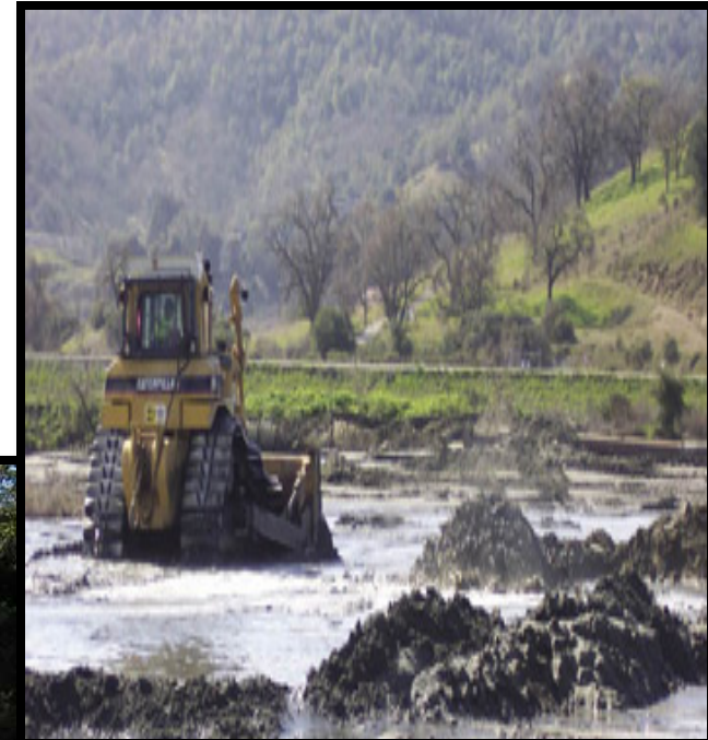
e.g., dredge and fill
