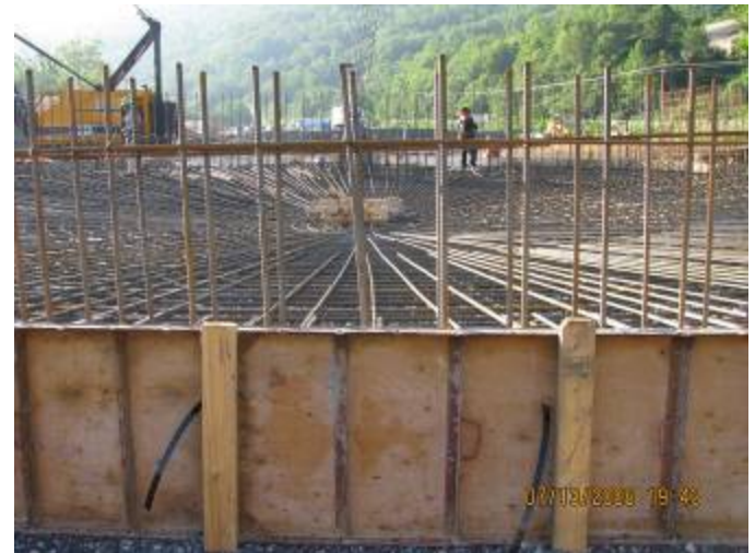
Georges Creek WWTP
