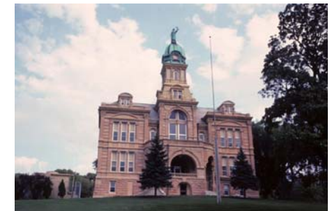
Blue Earth County Courthouse Mankato, MN
