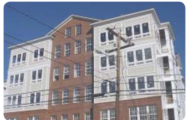
The Sierra under construction
